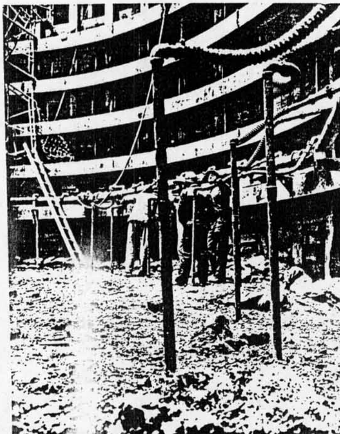
WCC Photo. SITE 8. BEHARR. Closeup view of well point system. Ladder and sectional scaffolding provide access to surface.
