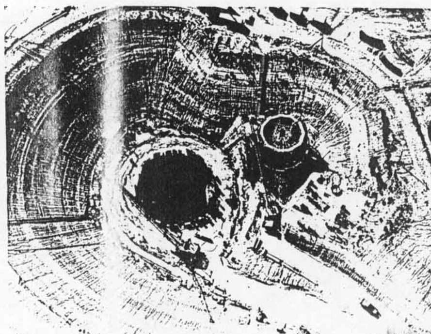
#41304. SITE 8, SEWARD. 11 Oct 60. Aerial view looking west. Note sheet piling around cilo. Work platform is in place around top of LCC in preparation for wall pour.
