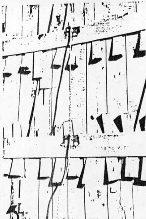
#C-7. Nov. 60. Close-up of ring beam structure shows manner in which oak wedges were used to secure the oak lagging behind the ring beams. Wedges were held with 50 & 60d nails. Note grounding cable attached to ring beams by exothermic welding process. Grounding lug at lower left. Wedges typical all sites using lagging.
