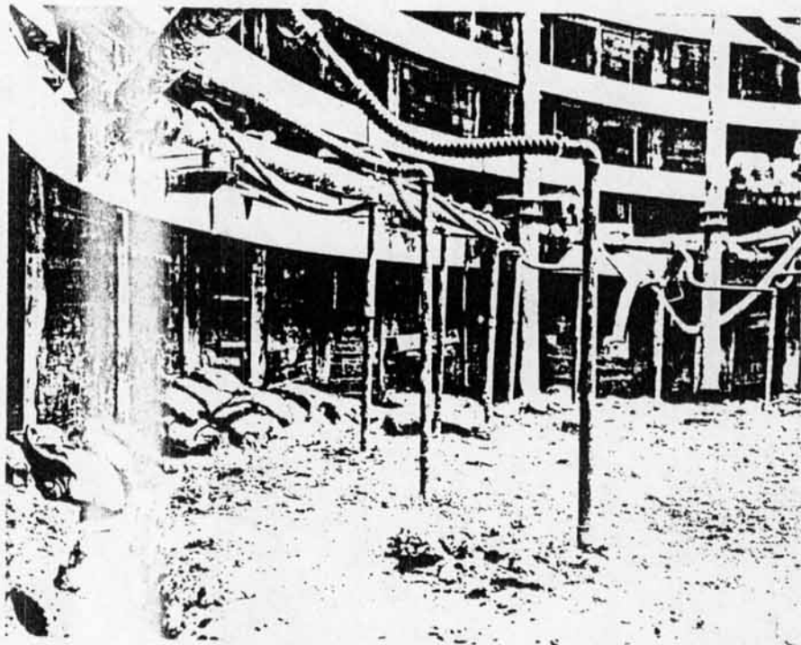
Photo. SITE 8, SEWARD, NEBRASKA. Shows closeup of well points and flexible connections to manifold.
